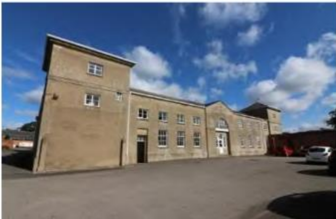
South Elevation – facing north elevation of Hall
