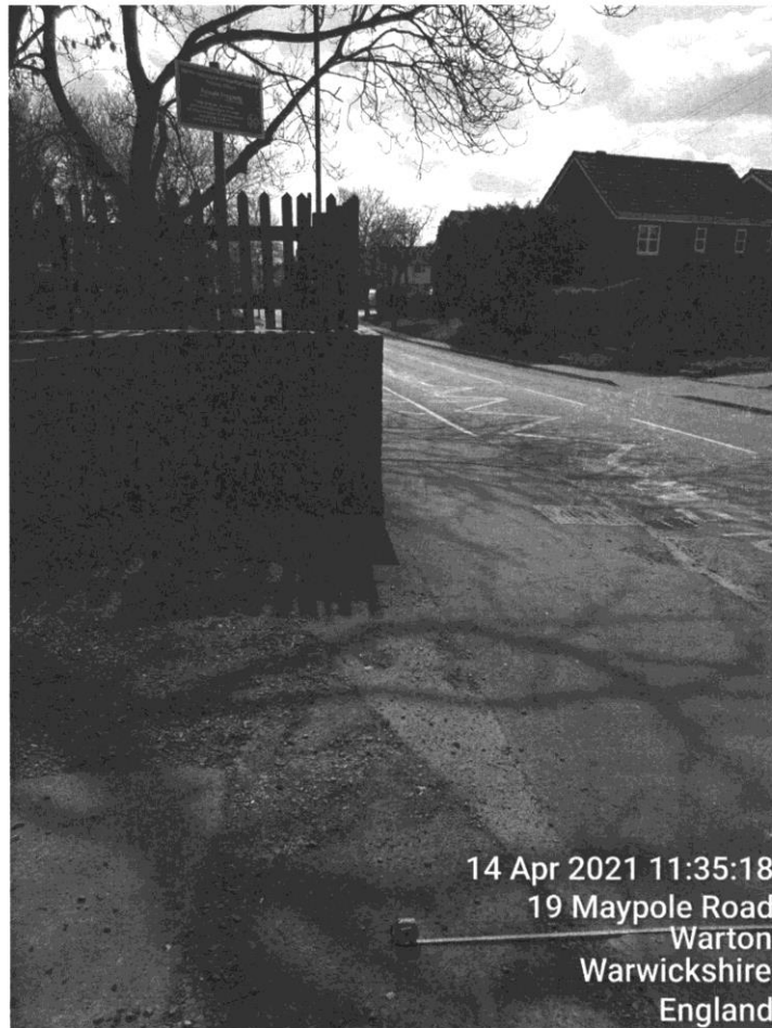
Left Hand Visibility – Photograph taken 2.4m back from the near edge of the carriageway (24.325m visibility set against a requirement of 43m)
