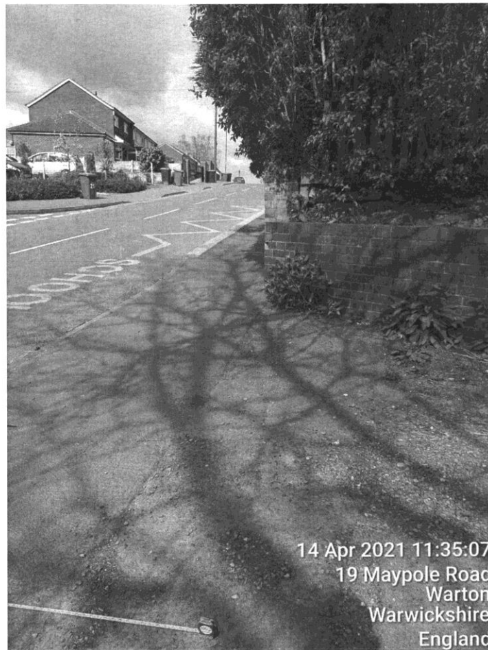
Right Hand Visibility – Photograph taken 2.4m back from the near edge of the carriageway (43m visibility achievable set against a requirement of 43m)
