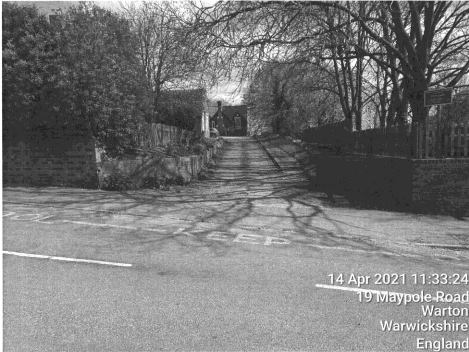
View of access into the site – photograph taken on the opposing side of Maypole Road
