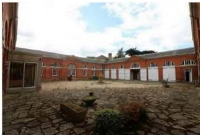
Courtyard north east
