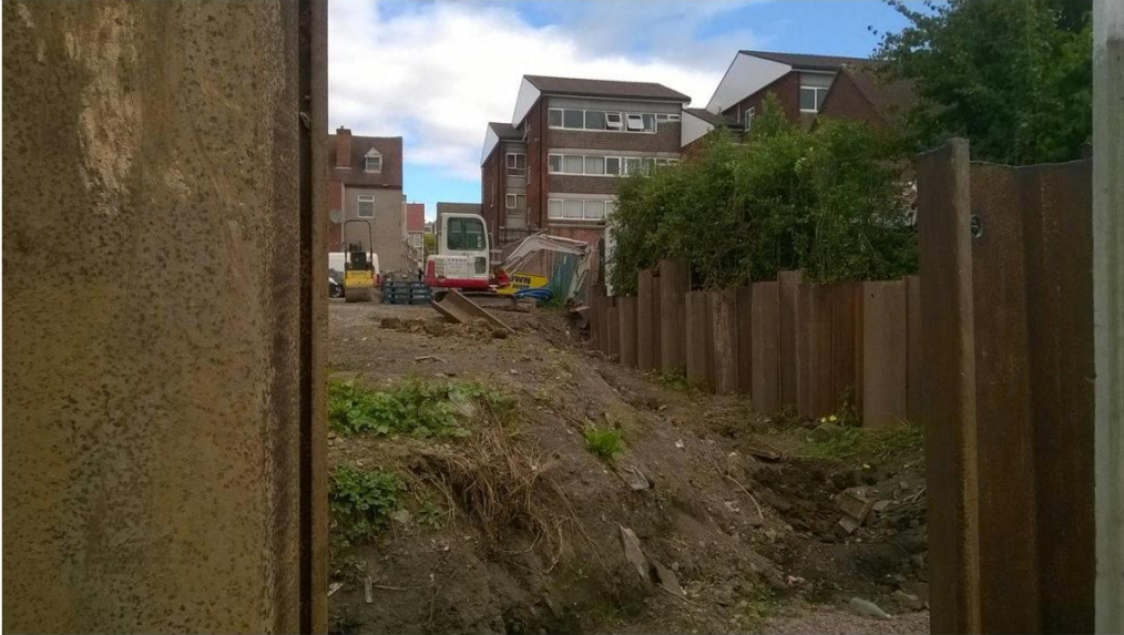
Photograph looking north towards Coleshill Road – Chancery Lane on right during development
