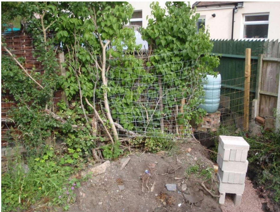
Photo taken from corner of boundaries of 9 & 11 Chancery Lane is the lowest point of the development site . Stream has now been piped in where the breeze blocks are stacked
