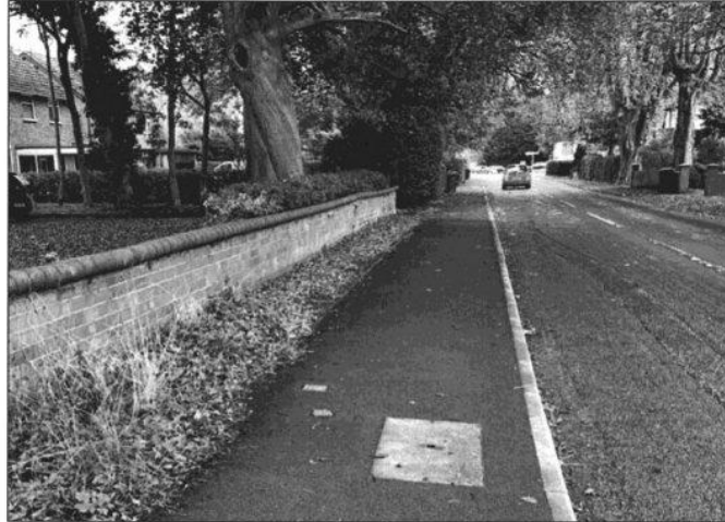
Photograph 4 – Existing highway verge
