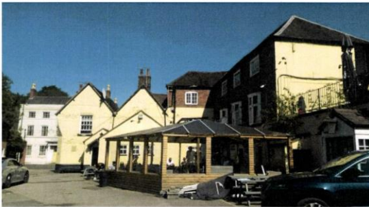
VIEW FROM CAR PARK (AUG 2022)
