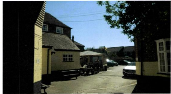
VIEW FROM CAR PARK ACCESS (AUG 2022)
