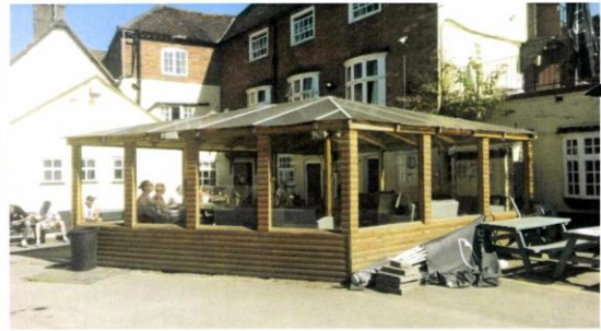
VIEW FROM CAR PARK (AUG 2022)
