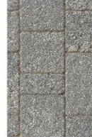
Permeable block paving
