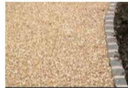
Bound gravel with granite sett edges
