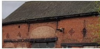
Brickwork details on existing farm buildings
