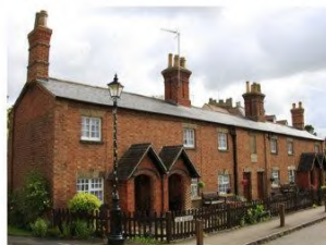
The Square, Dunchurch Red brick, pitched roof porches, prominent chimneys
