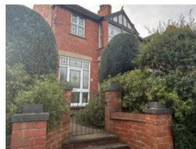
Low red brick walls, with grey brickwork coping in Atherstone conservation area
