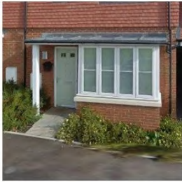
Porches combined with bay windows. Stone lintels.
