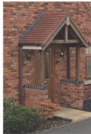
Porch on New Street using clay tiles and
