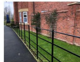
Estate style railings with brick garden wall
