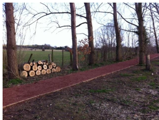
Habitat pile construction at Abbey Green Park © Alexis Evans (WWT)
