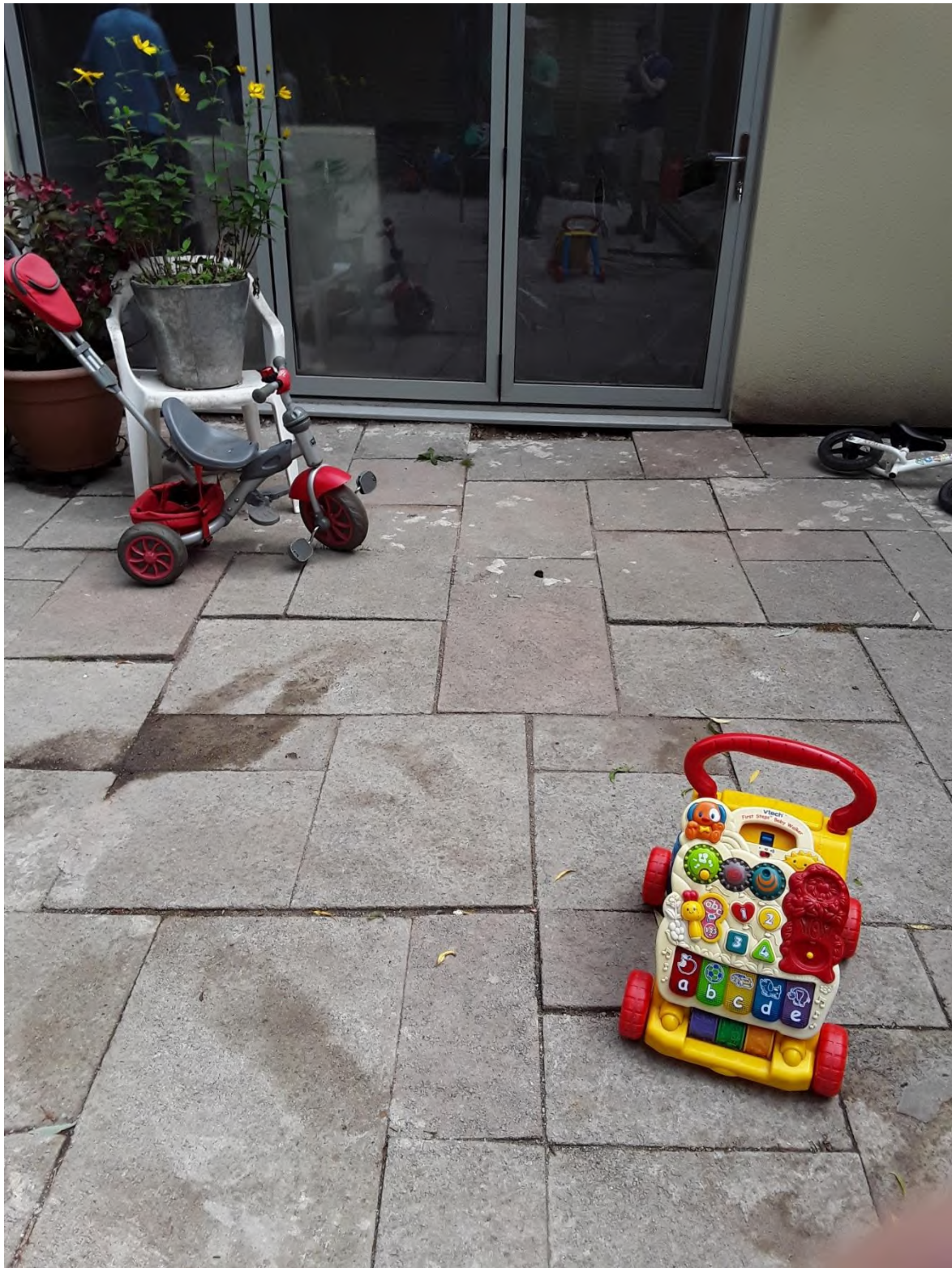
Image 12 – Showing patio area in relation to existing door way. Levels will need to be reduced
