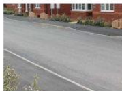
Tarmac roads and pavements
