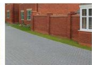
Brick garden enclosure
