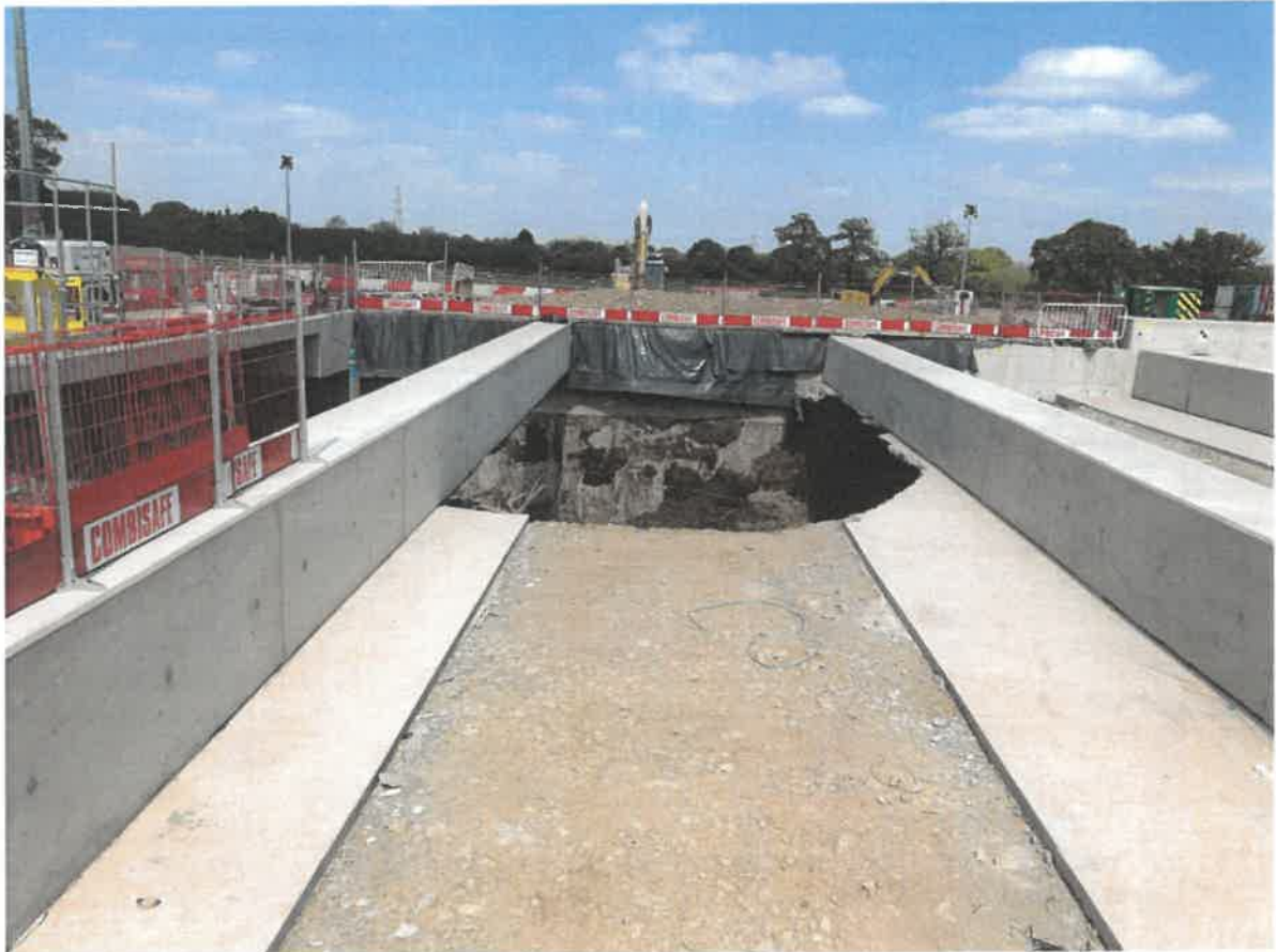
View looking northwards across the cutting, showing in-situ concrete props running between the northern and southern retaining walls and the partial excavation of the ground between a pair props
