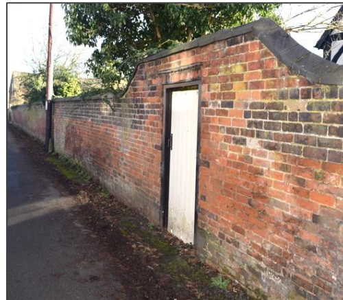
Tall brick wall on Old Church Road, incorporating a doorway and using a blue brick coping.
