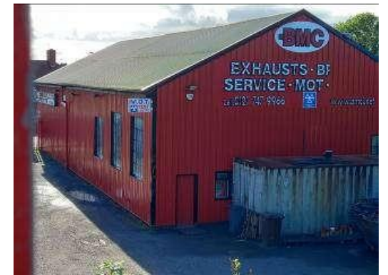
Industrial unit at Marsh Lane
