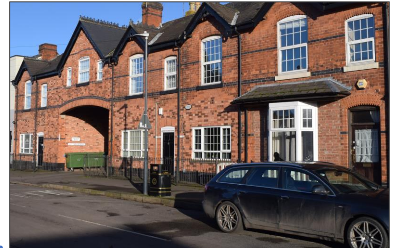
Replacement materials and style at 3-11 Coleshill Road
