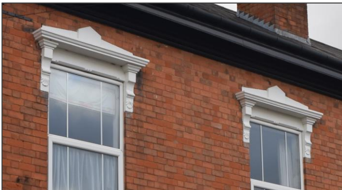
Good examples of stone window lintels at New Road.
