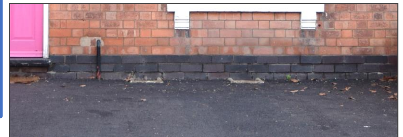
Raised ground levels at 2-12 Vicarage Lane
