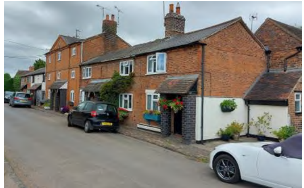
The row of former farm and estate workers' cottages at Caldecote Lane.
