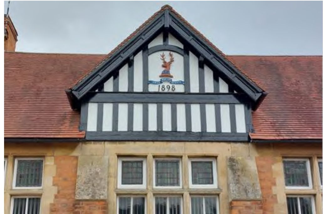
Figure 3.3: Village hall gable
