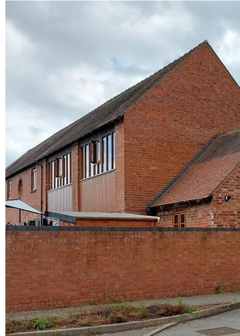
This barn range at the Courtyard is built of English bond brickwork, giving its walls a very solid appearance. The later single storey extension and boundary walls are of different brick laid in different bonds, but the use of red bricks and red clay roofs unites the new and old.
