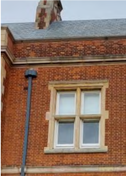
Detail of Caldecote Hall. The smooth stone dressings and Flemish bond brickwork form a visually pleasing contrast.
