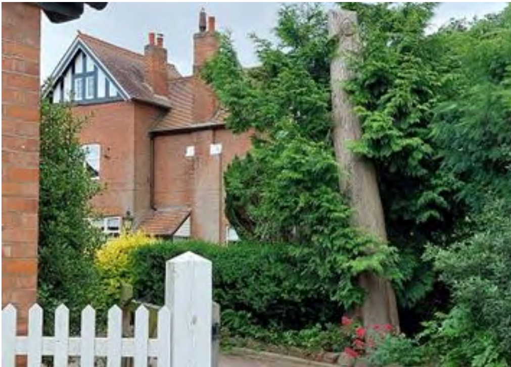
Figure A.7: The Beeches Farmhouse, Caldecote Lane
