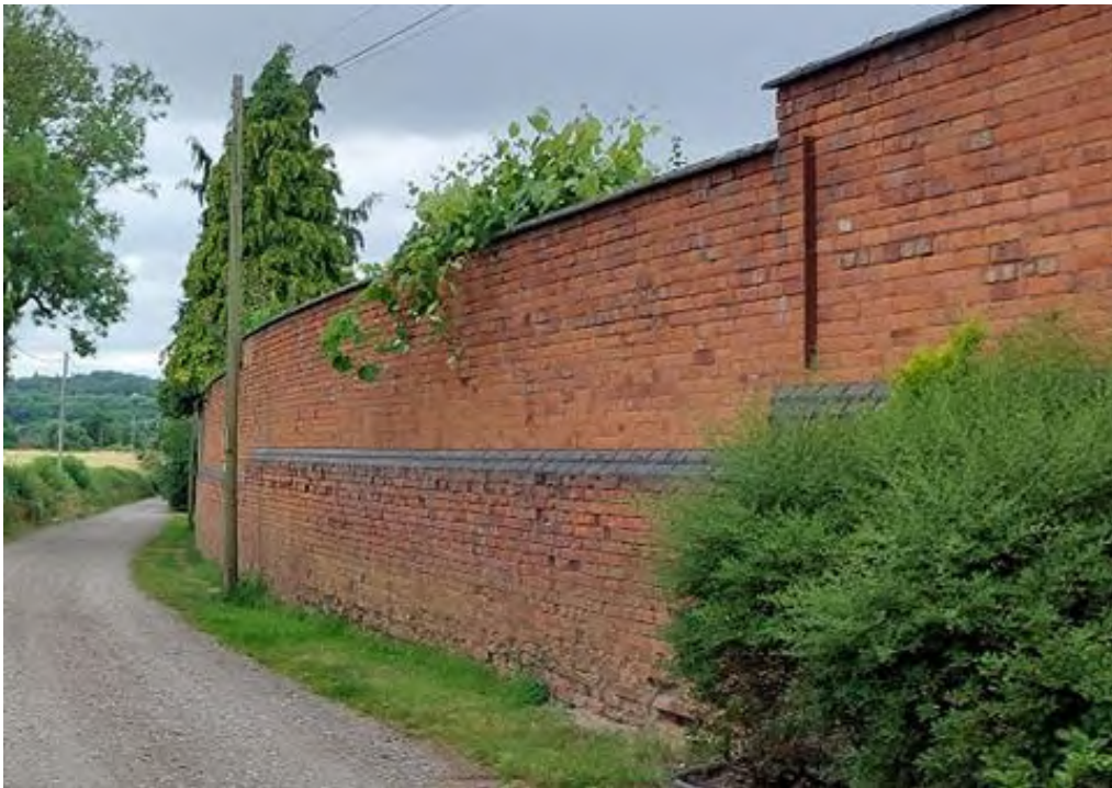
Figure A.5: The kitchen garden wall of Caldecote Hall as seen from Caldecote Lane
