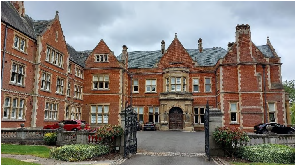
Figure A.1: Caldecote Hall principal entrance
