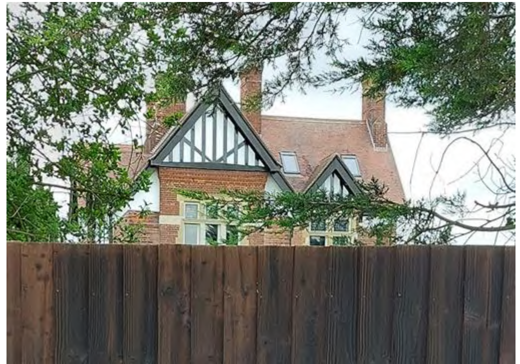
Figure A.8: The Grange, off Caldecote Lane
